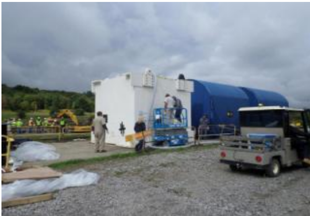
Melter Grouting Operations
